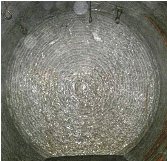
Fig. 10. View of excavated tunnel face using TBM (Vakola–vent hole tunnel section).
