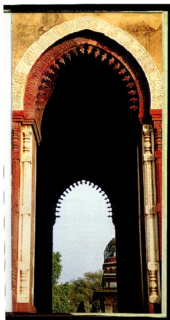
Fig: 22.5a A 'true' arch. The 'keystone' at the centre of the arch transferred the weight of the superstructure to the base of the arch.
