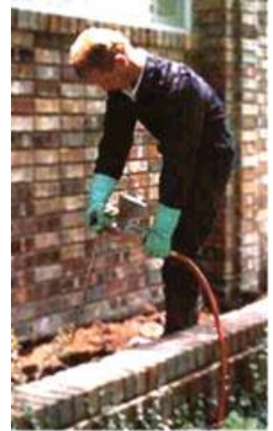
Liquid barrier application
