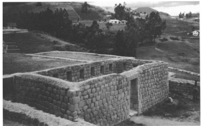
10 Inka, rectangular structure with trapezoidal portal and niches, Ingapirca, Ecuador, 1475-1530 (photograph by the author)
