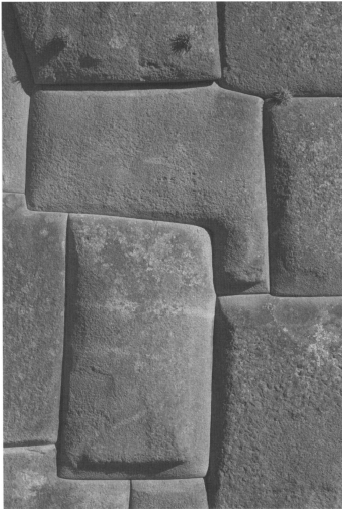
15 Inka, uncoursed masonry, Ollantaytambo, Peru, 1438-1530 (photograph by the author)
