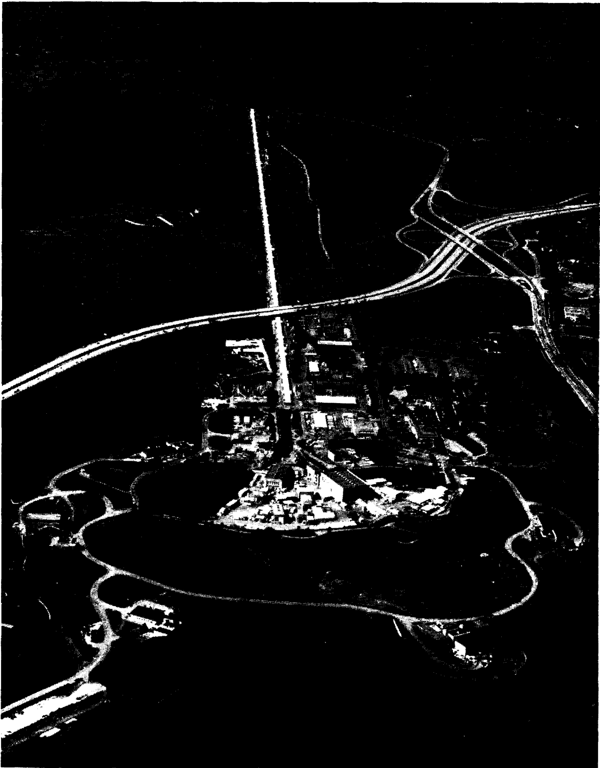
Figure I.1 The Stanford Linear Accelerator Center (SLAC). Electrons and positrons are accelerated down a straight tube 2 miles long, reaching energies as high as 45 GeV. (Photo courtesy of SLAC.)
