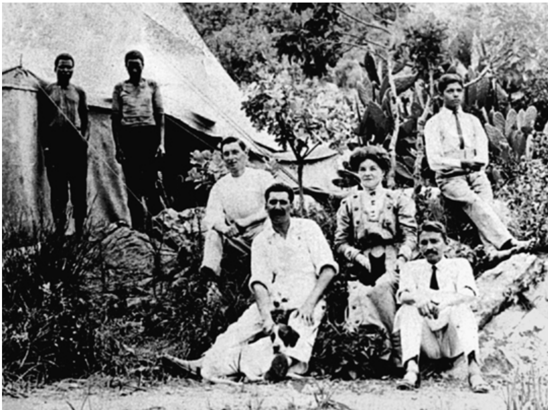
On the building site of Kallenbach’s new home (photo credit i3.1)
