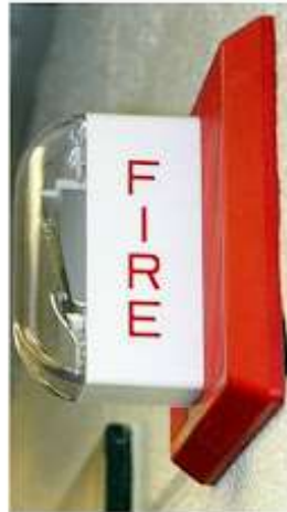
Fire Alarm Strobe
